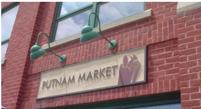
Figure 12: Example of a wall sign with external illumination, sized and placed to work with the architecture of the façade.
