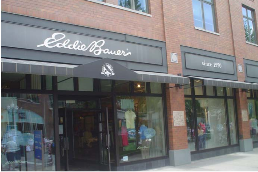
Figure 18: Example of an internally illuminated cabinet sign which has been recessed into the façade so as to appear to be part of the architecture. The white lettering is the only portion of the sign which is illuminated at night, while the remainder of the background is black to blend with the dark panels of the façade.
