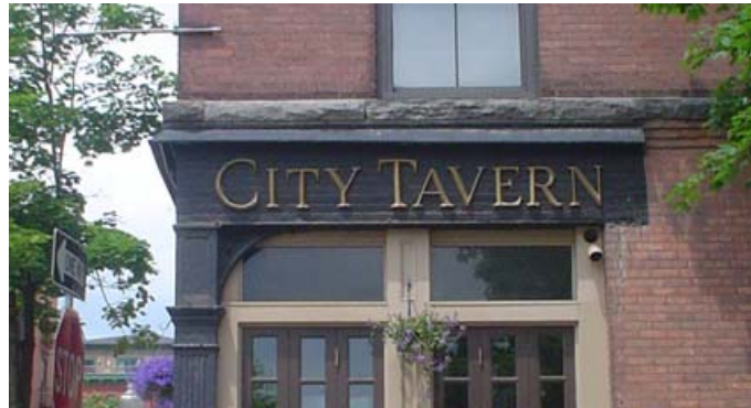
Figure 11: Example of surface applied channel lettering which has been sized and placed to work with the existing architecture of the façade.
