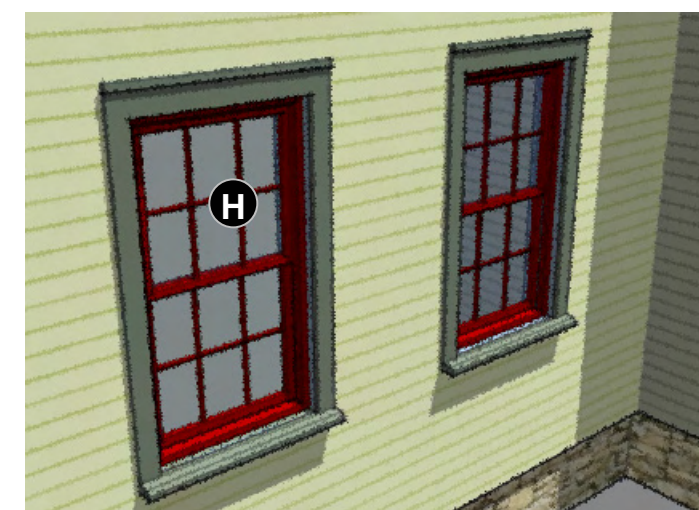
Fig. 4: Standard double hung divided lite windows with wood trim. The bold wood trim helps to give added depth and shadows to the window openings which you do not get from the thin edges of typical vinyl siding trim.
