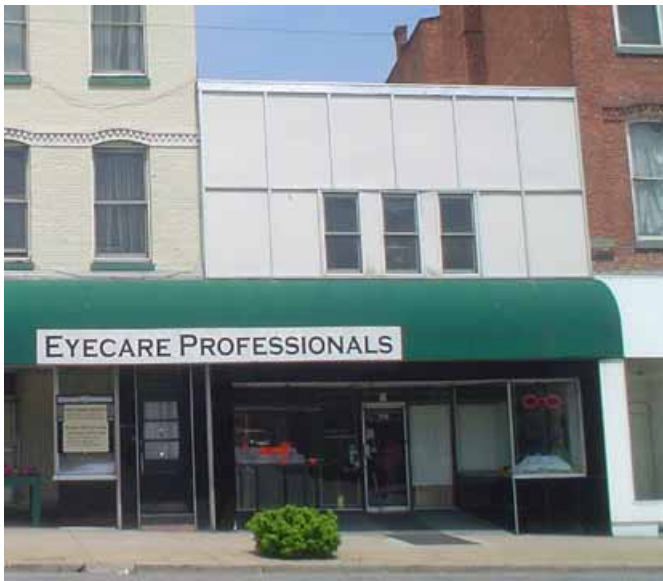
Concealing original façades behind newer materials often results in a loss of architectural detail, scale and character.
