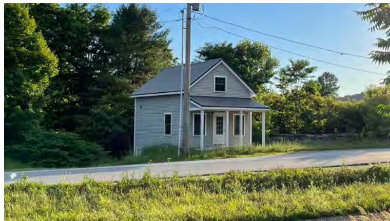
▲ Duquette Property. Non-contributing structure, recently rebuilt to replace 1910 structure lost in Dutchies fire. Currently vacant.
