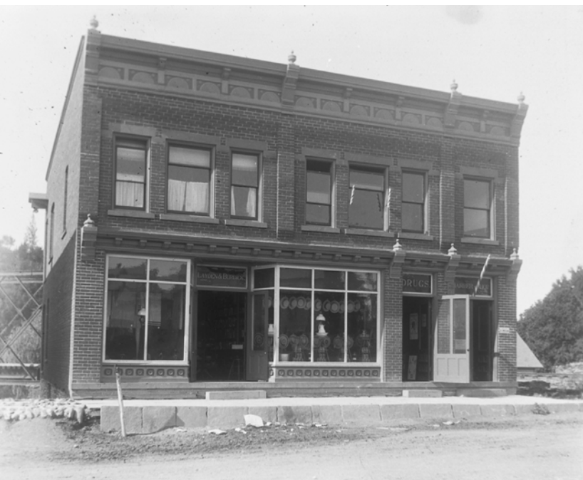
▼ Layden & Burdick General Store. Once home to the local Pharmacy and Soda Fountain, today serves as community space and apartments, known as the “Celery Compound” in reference to the antique advertisement painted on the west facade.
