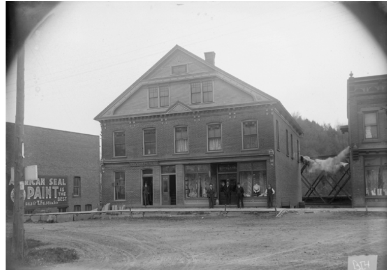
▲ Rising & Nelson. The Rising & Nelson Roofing Slate building, with Copeland Boots, Shoes, Groceries and Dry Goods Store, today serves as the Post Office.
