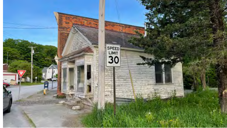
▲ 13 Egg Street (Antiques Store). Contributing structure circa 1910 store, featuring original storefront design. Currently vacant. Owner would like to rehabilitate building and turn into small store serving community and rail trail users.
