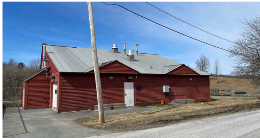
▲ Wastewater Treatment Plant. Currently operating well under capacity, this facility represents growth potential, but needs new users to help bring down operational costs.
